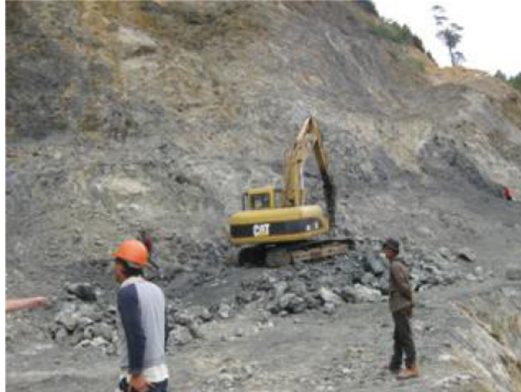
Figure 4-2: Corner of the Mining Area within the Mine
